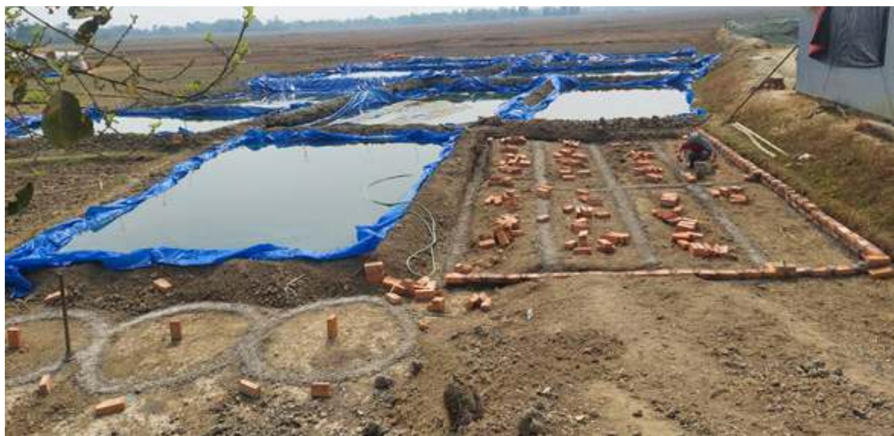
Construction of small-scale fish hatchery unit
